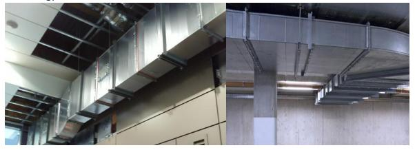
"SFRD" Fire Rated Ductwork has passed the stability, integrity criterion for up to 240 minutes & insulation for up to 14 minutes as per BS 476:part 24:1987 and it has also passed the integrity, smoke leakage criterion for up to 240 minutes & insulation for up to 14 minutes as per EN 1366:1:2014.
