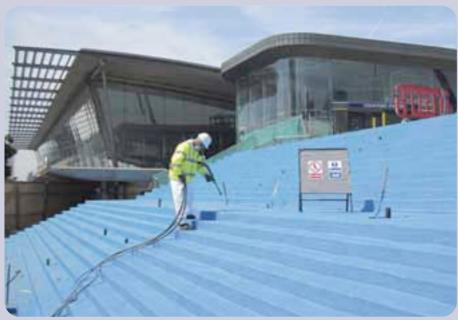
Blueshield PmB is a rapid curing, two part, spray applied, durable corrosion protection and waterproofing material. The high performance system is 100% polyurethane, containing no fillers or additives and is VOC free. Once applied, Blueshield PmB has exceptional bond strength to all commonly used substrates, has excellent crack bridging capability, a life expectancy in excess of 30 years and holds British Board of Agrément approval.
