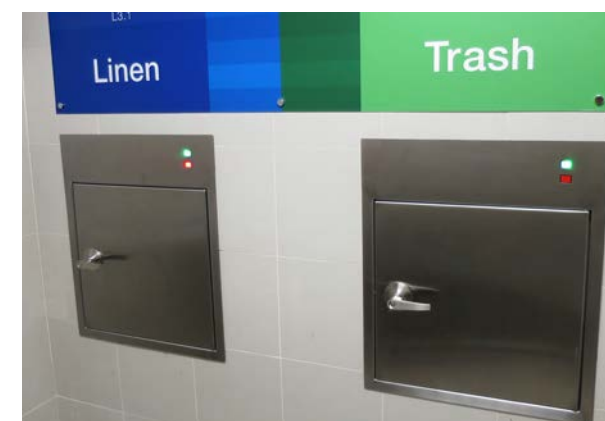
General waste and soiled linen have separate inlets but can be transported through the same pipe.
