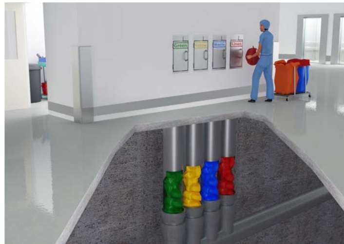
One pipe solution with separate wall inlets, chutes and storage valves for each material.
