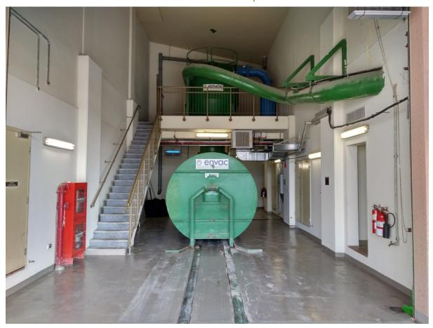
Envac's system consolidates waste into one container which is removed and replaced once per week. When compared to conventional waste collection practices, which require daily collection, the use of Envac's system results in an 80% reduction in waste collection vehicle trips.
